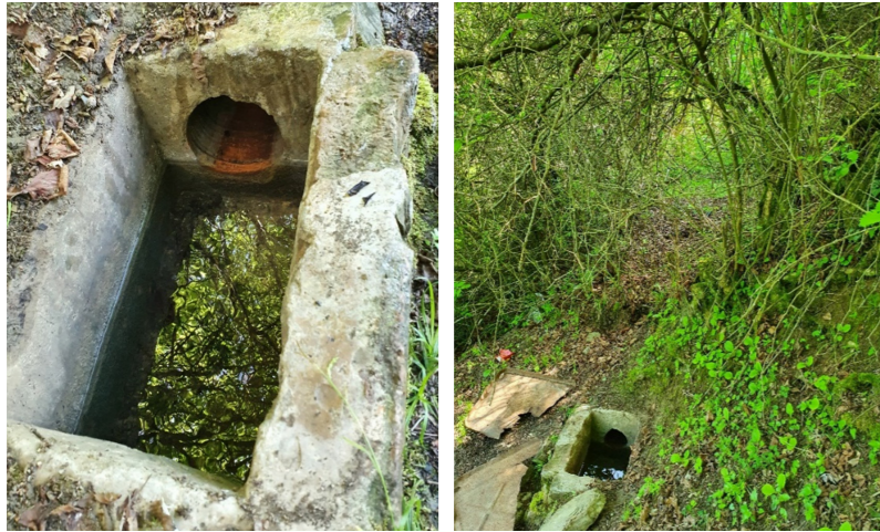
The Tajliq Su water pipe brings water to the Ganjali part of Sheki. Local residents estimate that it is at least 300 years old. 2021 © Rovshan Abbasov
