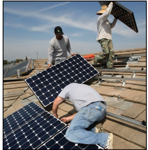
Workers install solar panels on the roof of a house.
