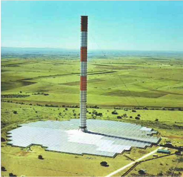
Fig. 3. A view of the Manzanares Solar Chimney Power Plant
