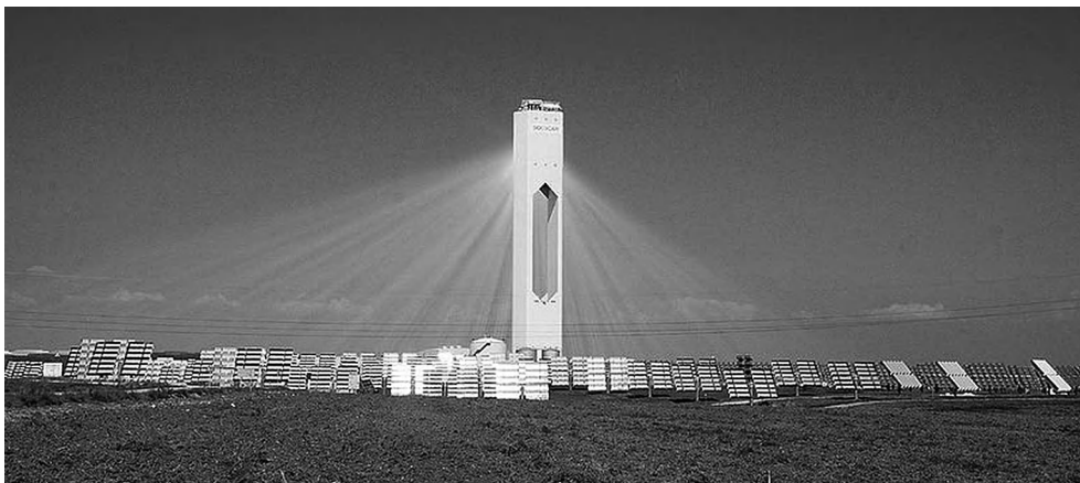
Figure 2.10 Solar power tower in operation, note the highly focused light near the power towers collector.
