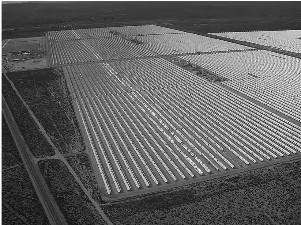
Figure 2.7 SEGS parabolic trough power plant in Southern California.
