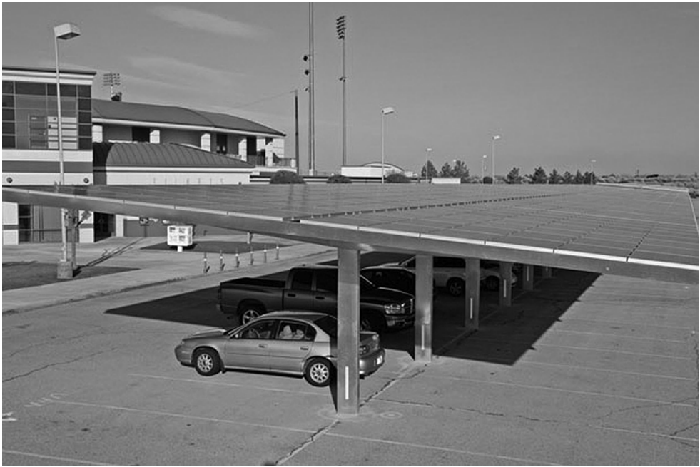
Figure 9.8 Carport in a parking lot (Courtesy: Baja Construction Co. Inc).
