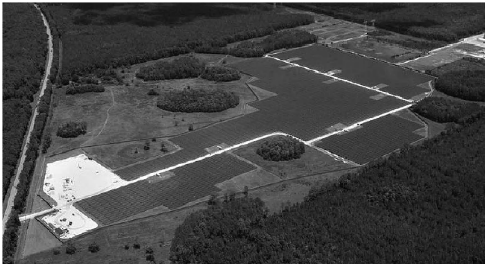
Figure 8.3 View of Jacksonville Solar 15 MW solar project area and wetland areas. Note how the wetland areas were avoided in the final site layout (Collins, 2010).
