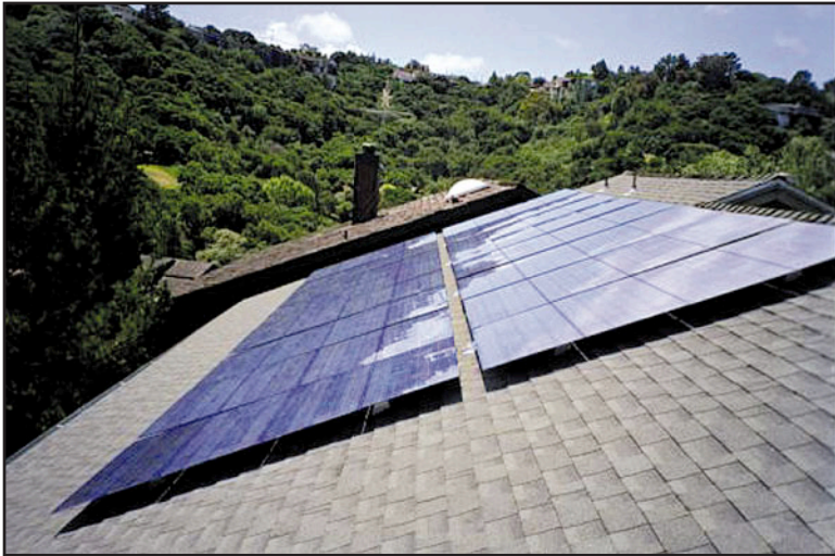
Figure 9 — Fixed roof mount
