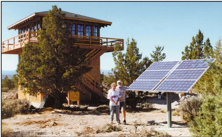
Figure 8 — Tracking pole mount
