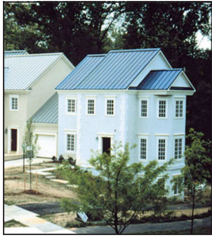
Figure 12 — Roof integrated thin-film modules
