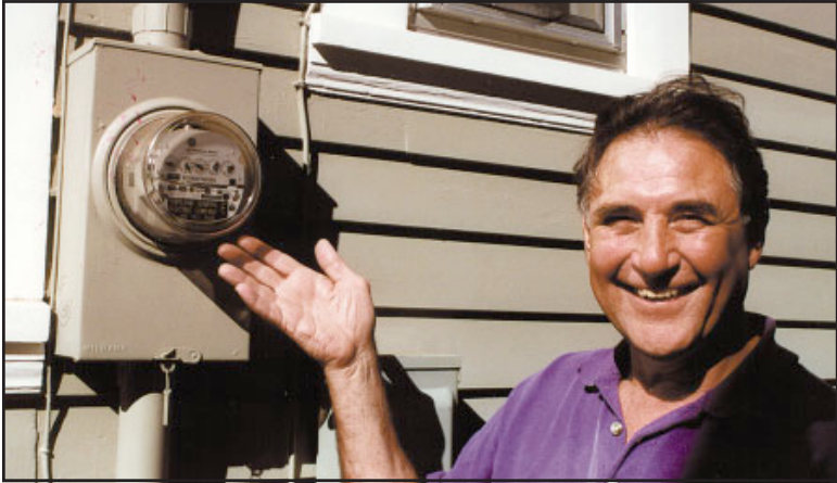
Figure 18 — With net metering, surplus power spins the meter backward.
