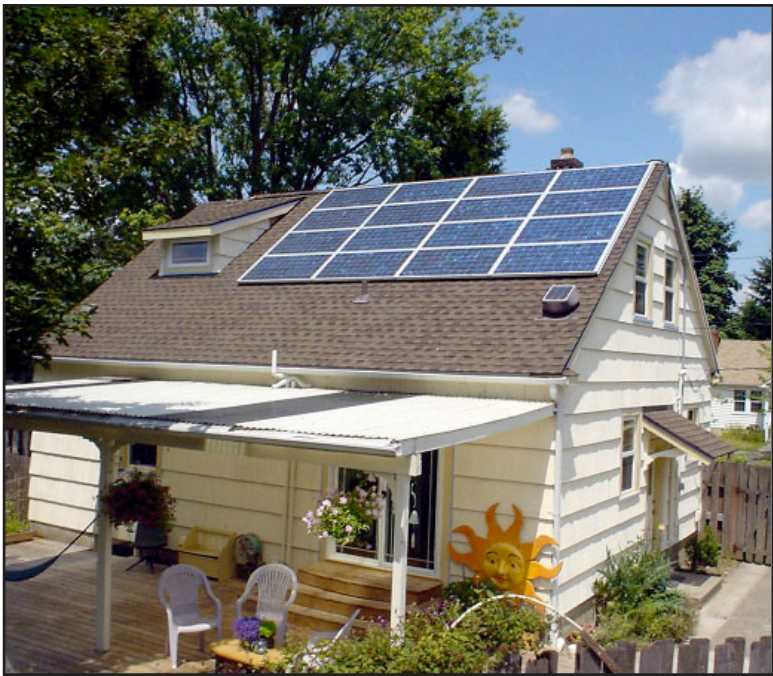
Figure 1 — Solar powered 1929 home in Salem
