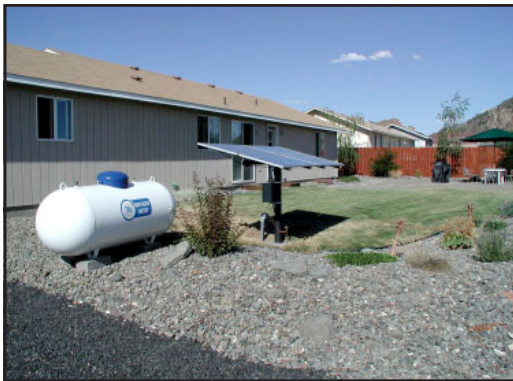
Figure 10 — Fixed ground mount
