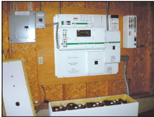
Figure 21 — Power panel with battery box
