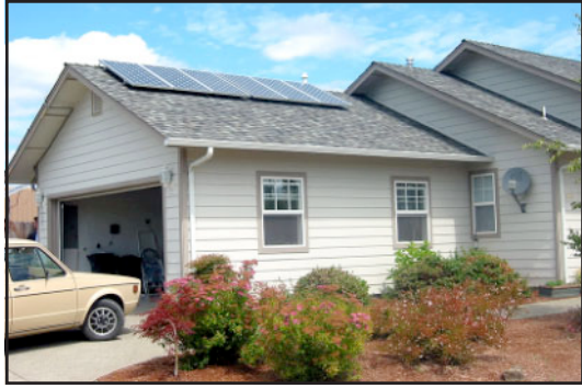
Figure 14 — Renewable solar energy on a Grants Pass home
