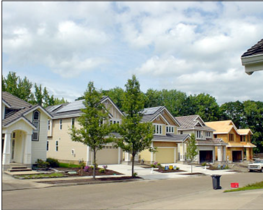
Figure 16 — Four solar-powered homes being built in Corvallis
