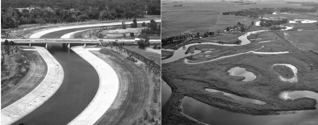
Photos 3.2: Highly channelized red Rouge River Dearbon for flood control purposes source USACE; Photo 3.3 Riverine Wetlands in Northwest Iowa, Source Lynn Betts.
