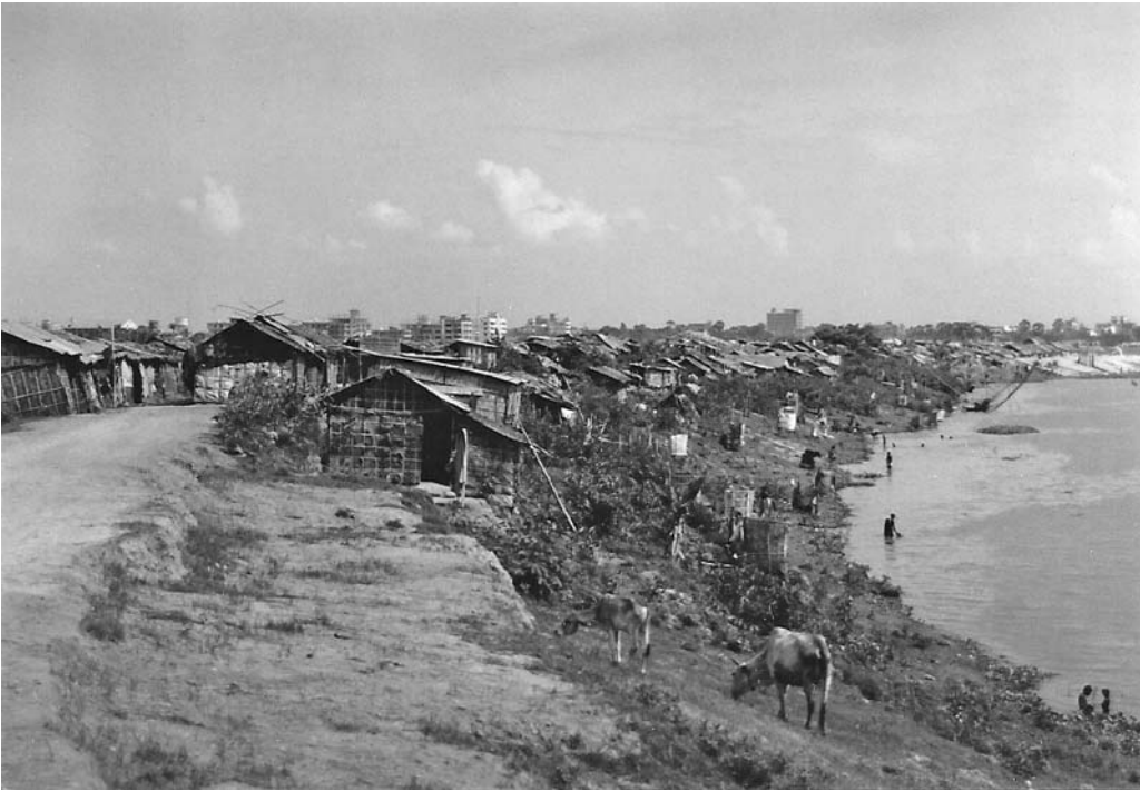
Photo 3.17: Multipurpose embankment with erosion. Source: Alan Bird
